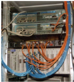
The FC network runs in conjunction with a FC-switch.
